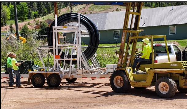
Our field technicians loading a roll of HDPE.
